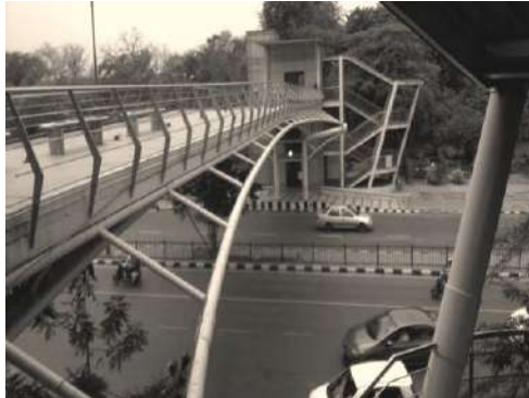
Pedestrian Bridge, New Delhi
